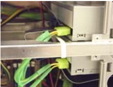
2.3.Connect 4-pin cable connectors from power supply to all 3.5" and 5.25" devices.
